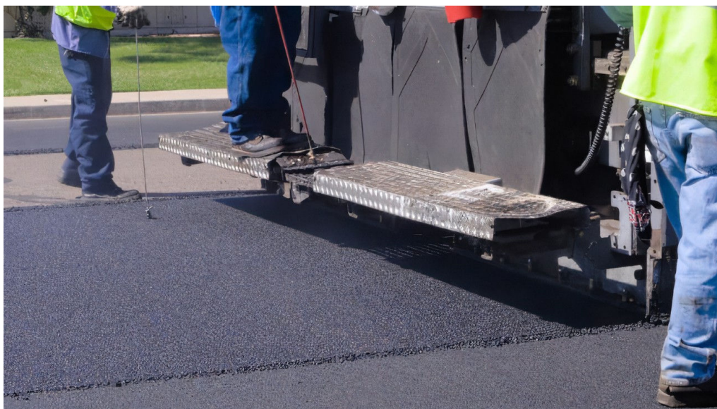
Figure 1: Ultra-Thin Bonded Wearing Course being laid 1
