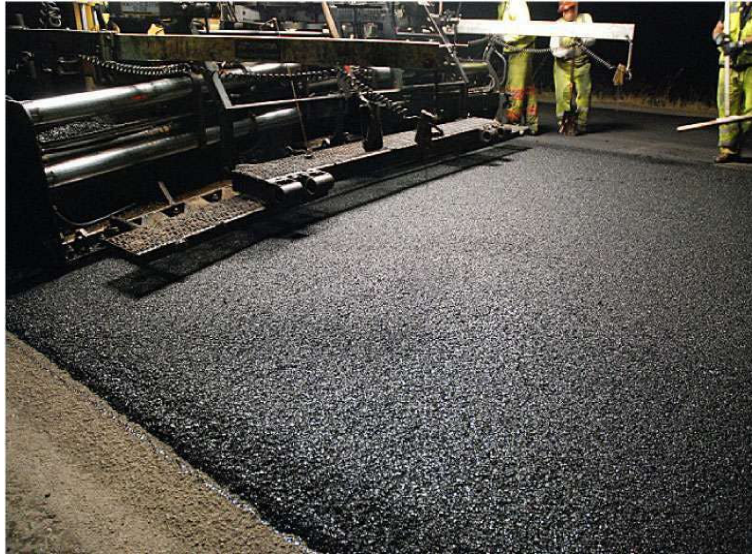
Figure 1: Open Graded Friction Course paving process.
